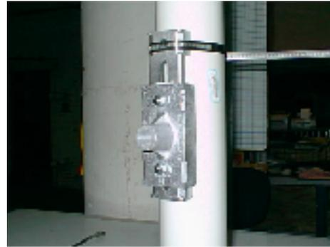
Wrap the first steel band around back plate at top and tighten down. Remove duct tape and place rod plate over stove bolts.
