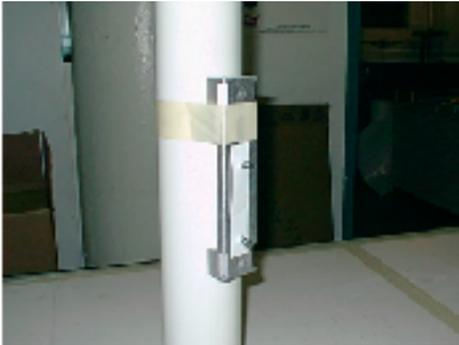
Place bracket plate at desired height on light pole and duct tape to pole to hold in place.
