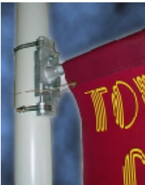
Slide banner on to bracket arm at top and loop wire or electric ties through grommets and around lightpole to insure banner will not slide off of arm.
